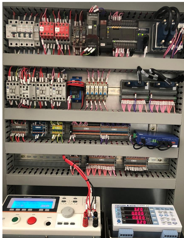
Electrical Test Station
